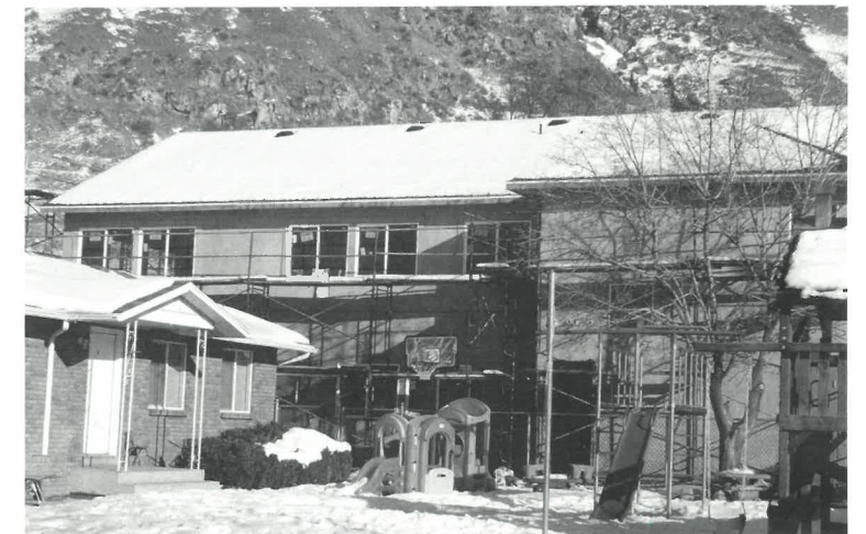
House of Hope (Provo) new addition during construction this winter.
