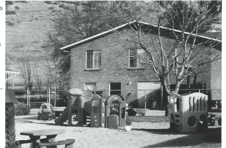
Treatment Building: View of where new wing will be built
